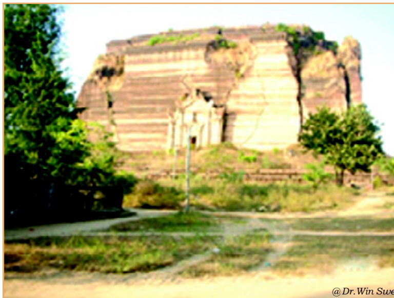
Mingun Pagoda, severely damaged by 1839 Ava earthquake, before its completion of construction and again by 1956 Sagaing earthquake.
