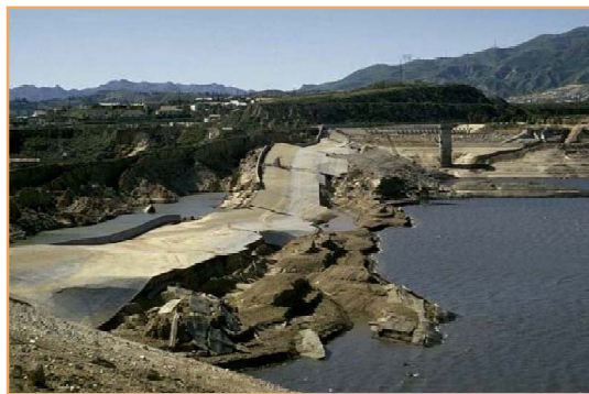
Lower Van Norman Dam experienced widespread liquefaction and major slope failures during the 1971 San Fernando Earthquake
