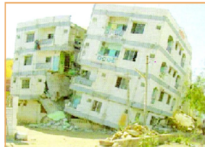
Collapse of buildings during 2001 Bhuj (India) Earthquake
