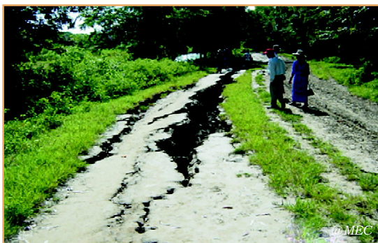
Fissures formed during 2003 Taungdwingyi Earthquake, central Myanmar
