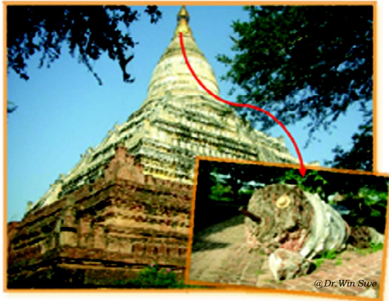
Top of the pagoda shaken down by the 1975 Bagan earthquake, now lying down beside the renovated original pagoda.
