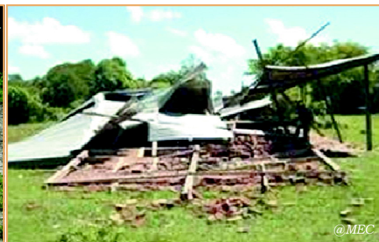
Collapsed primary school during the Taungdwingyi earthquake
