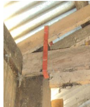
Metal tie between roof cords
