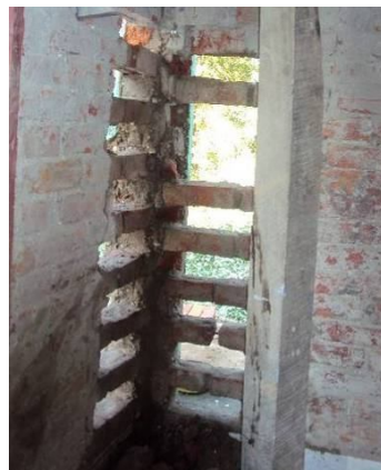
Open-up for corner repair
