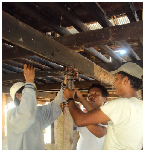
Leveling the floor girder
