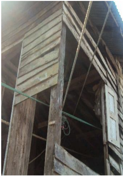
Pulling the building for verticality
