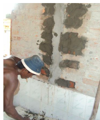
Plastering back stitching
