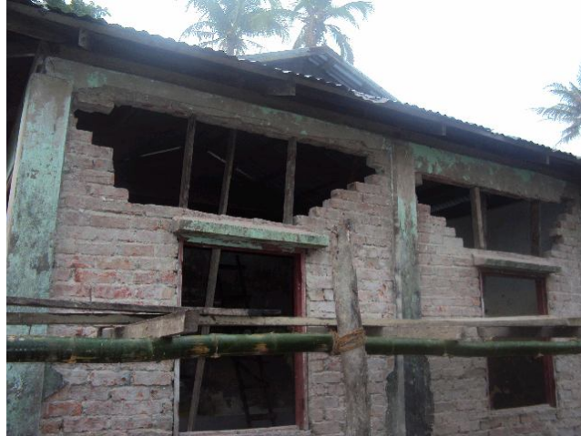
Removing loose bricks and plaster
