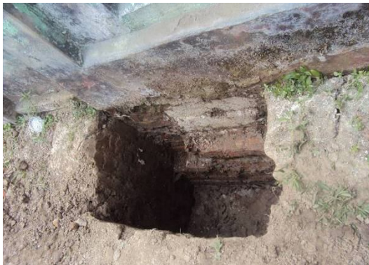
Preparation for additional column foundation
