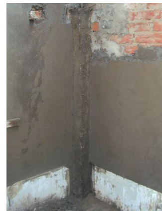
Concreting and plastering
