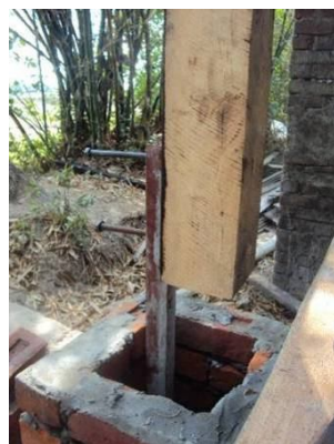
Replacing defected member
