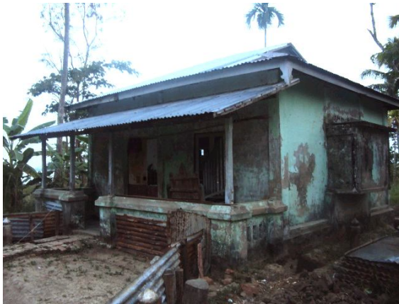
Assessing the building before retrofitting
