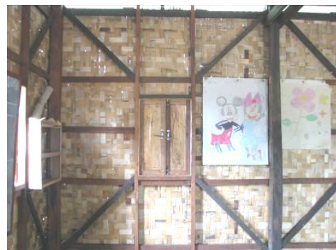
Bracing of a bamboo building
