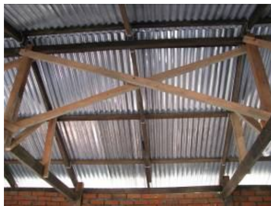
Vertical cross bracing between trusses
