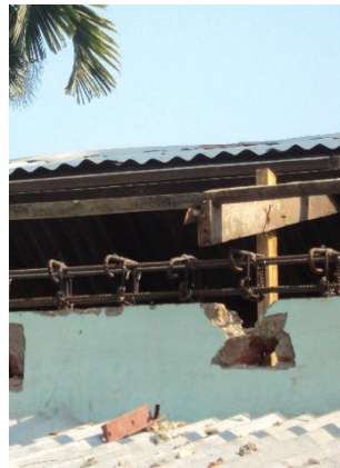
Preparing reinforcement for roof tie beam
