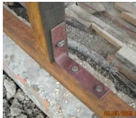
Sill and stud connection detail
