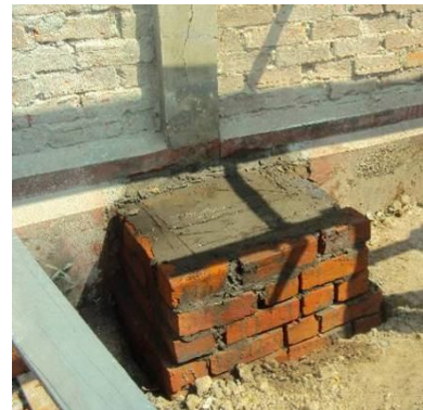
Making new brick foundation
