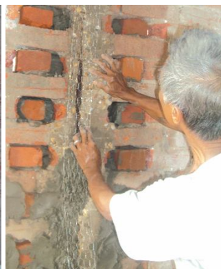
Installing Mesh
