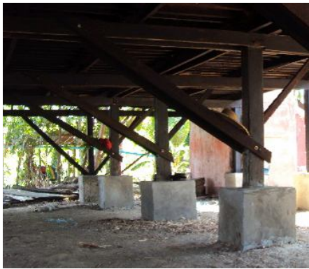
Providing Knee Bracing
