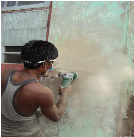
Removing loose plaster
