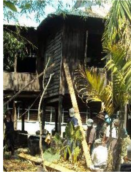
Shoring the building for verticality
