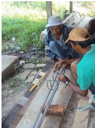
Preparing reinforcement for roof tie beam
