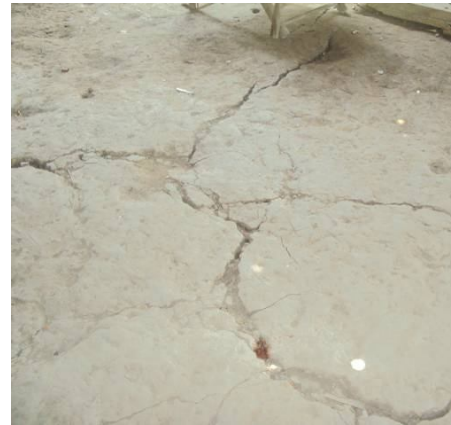
Floor cracks
