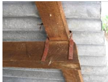
Metal tie between purlin and rafter
