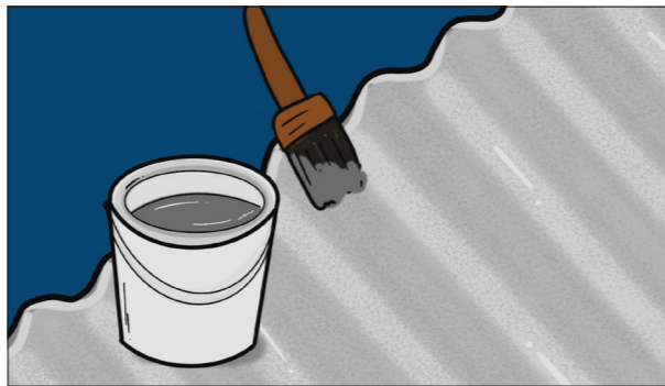
Photo showing the application of heat reflective coating on the iron sheet roofing
