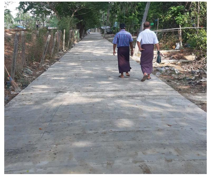
The purpose of upgrading basic infrastrucutre and services was to enhance accessibility to WASH and clean potable water sources. The project improved/ upgraded road segments to/ from water supply systems, improved drainage/ culverts alongside the roads, and installation of solar street lamps.
