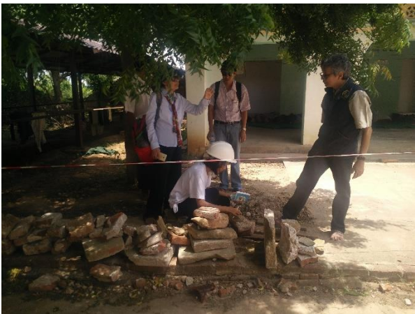
Figure 6: Post Earthquake Assessment after Chauk Earthquake
