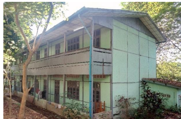
Figure 65: No sign of any distress
