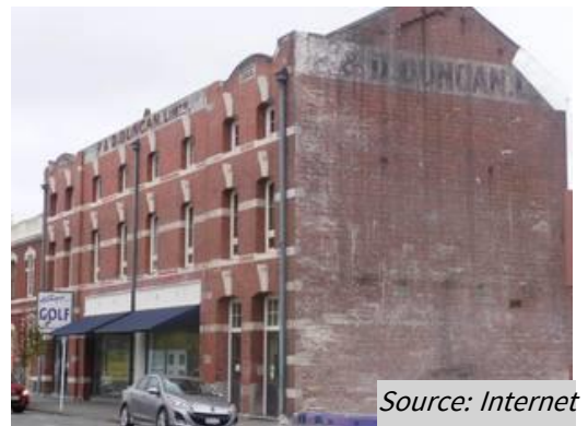
Figure 73: No sign of any distress
