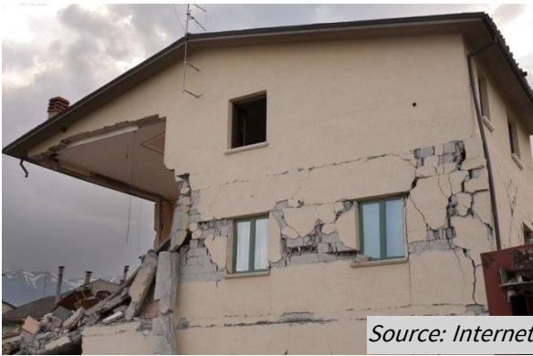
Figure 86: Partial collapse
