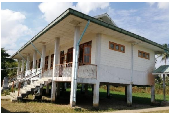
Figure 82: No sign of any distress
