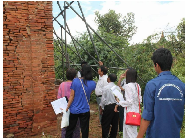
Figure 7: Post Earthquake Assessment of Temple buildings in Bagan after Chauk Earthquake
