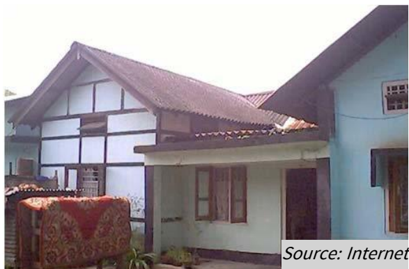
Figure 64: No sign of any distress
