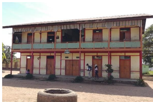
Figure 14: Brick Nogging building
