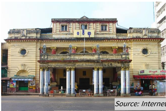
Figure 72: No sign of any distress
