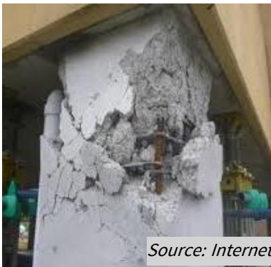
Figure 55: Reinforcing bars are exposed due to spalling of the covering concrete (Moderate)
