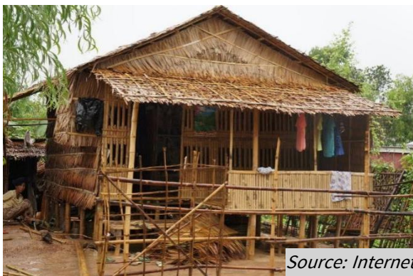
Figure 59: No sign of any distress (Bamboo building)
