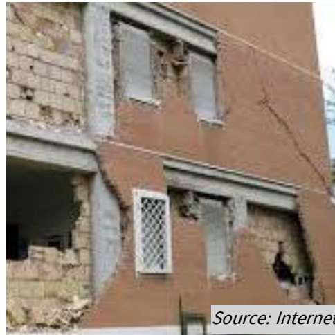
Figure 40: Infill walls, partitions
