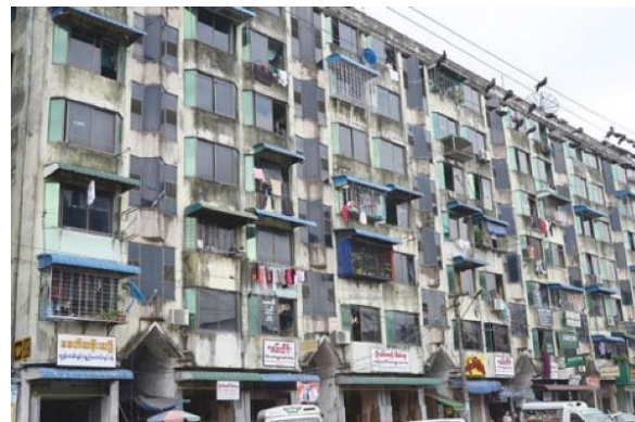
Figure 83: No sign of any distress
