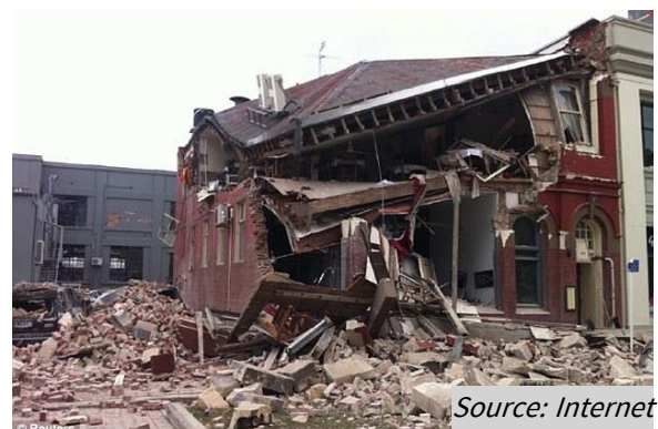
Figure 52: Partial Collapse (Severe)
