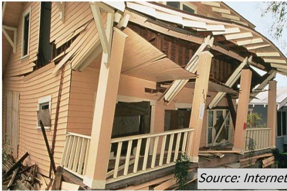
Figure 62: Partial collapse
